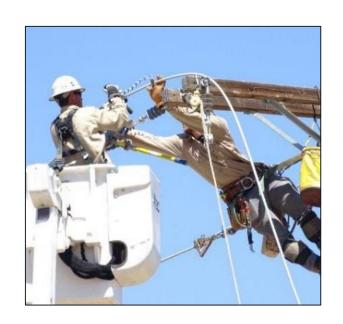
Insulation on wire prevents faults (tree limbs, windborne debris, metallic balloons, etc.) that can lead to ignitions
